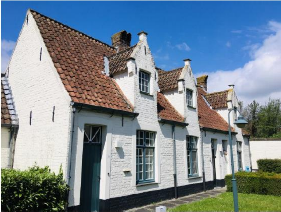
Figure 1: Building with 2 (out of 15) dwelling units
